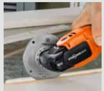
Cutting through nails on window bars.
