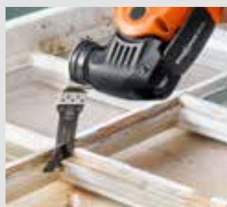
Restoring old windows.
