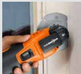
Cutting through metal bracings when dismantling old windows.
