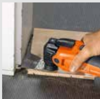
Work flush with the surface.
