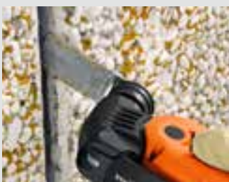
Roughening the mortar flanks before filling in again.
