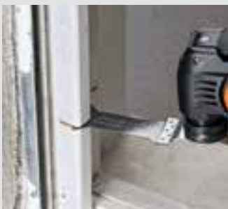
Cutting through window frames.
