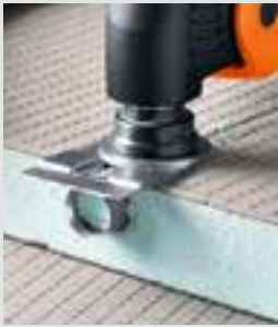
Cutting out channels for hot water underfloor heating.
