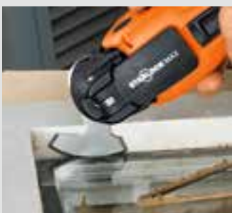
Cutting out putty-mounted insulation glass windows.
