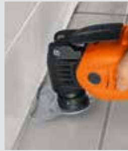
Removing elastic grout sealants.
