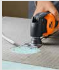
Preparing for electrical installation.
