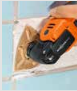
Sanding tile adhesive flush before filling in again.
