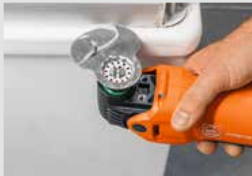
Remove joint fillers.
