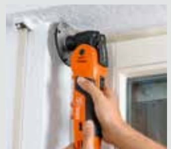
Cutting open covers on roller shutter cases.
